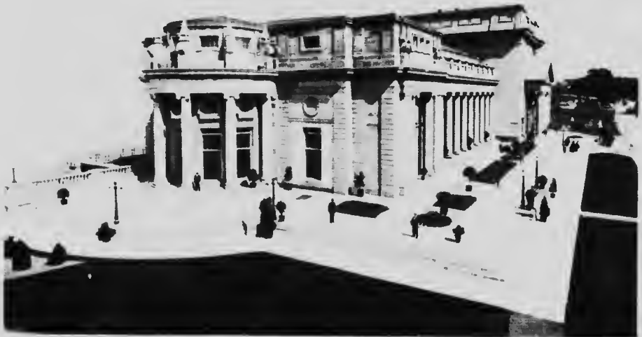
Power House, Electrical Development Company, Niagara Falls, Ontario.
