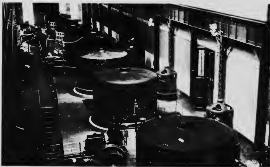
Power House of Electrical Development Company, Niagara Falls. Interior View.
