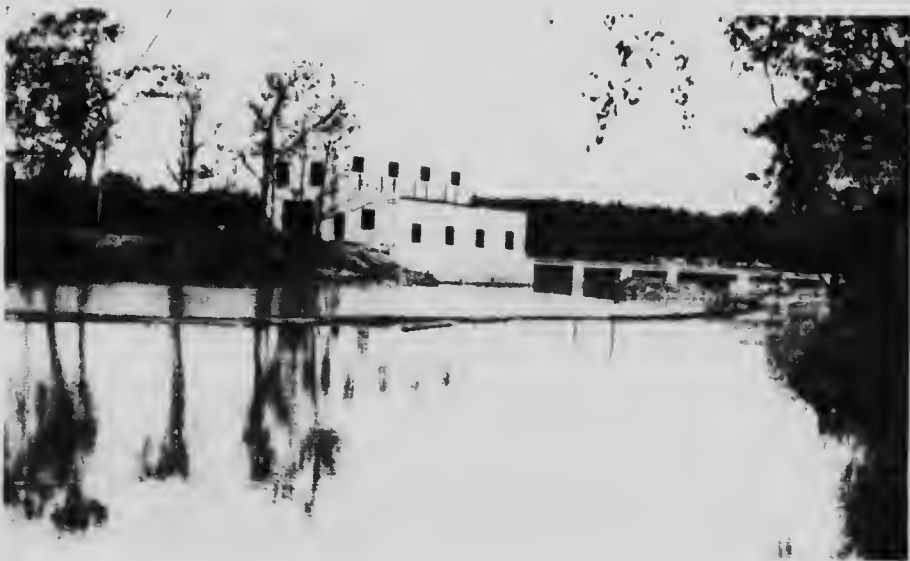
Waddell's Falls Development, Hydro-Electric Power Commission of Ontario.
