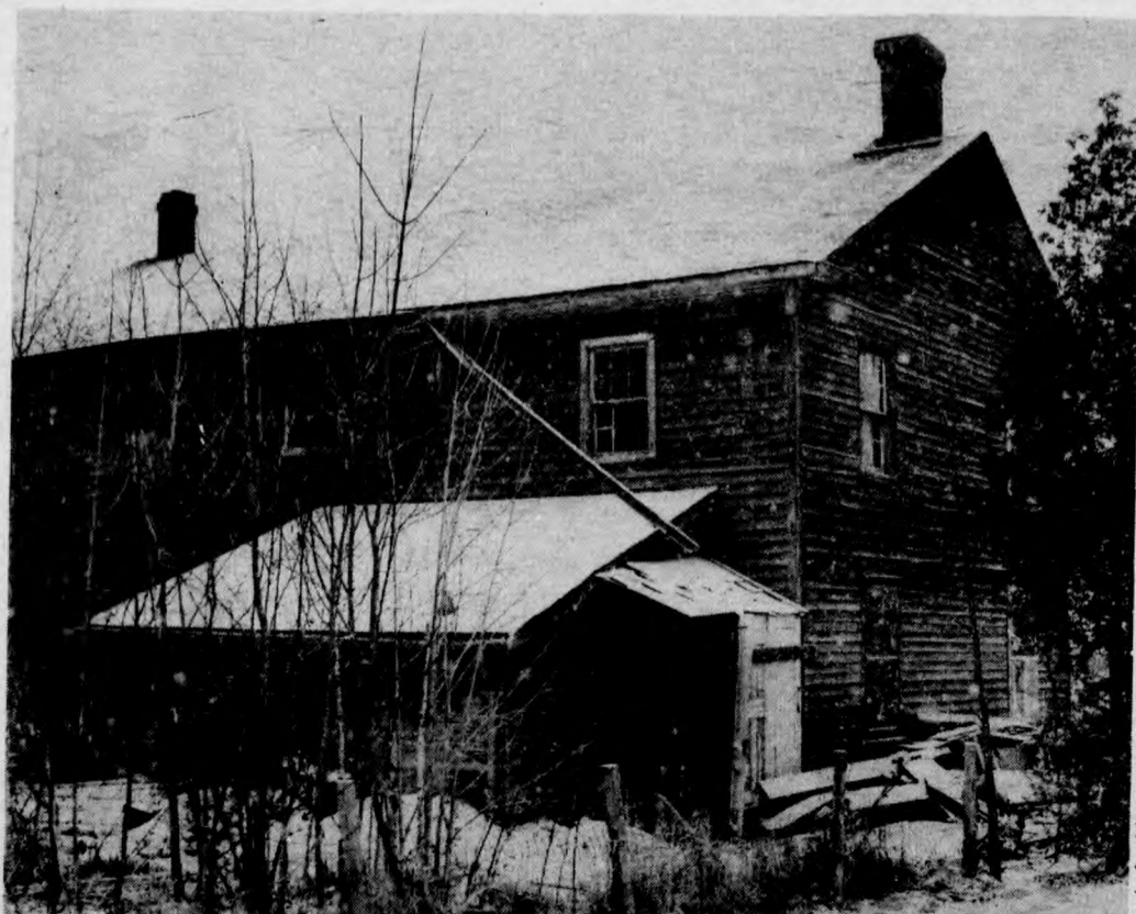
Green Bush Inn just prior to demolition.
