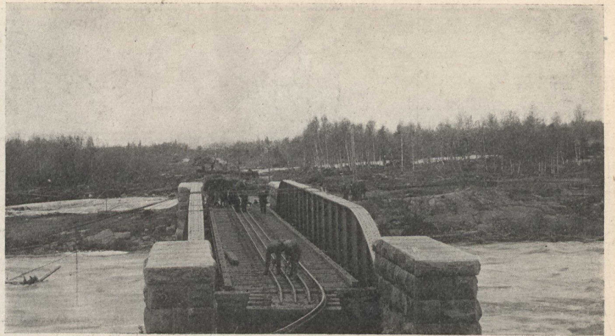
Looking west towards Port Arthur, showing where flood carried away track and road bed. Wires across bridge are from the power house.
