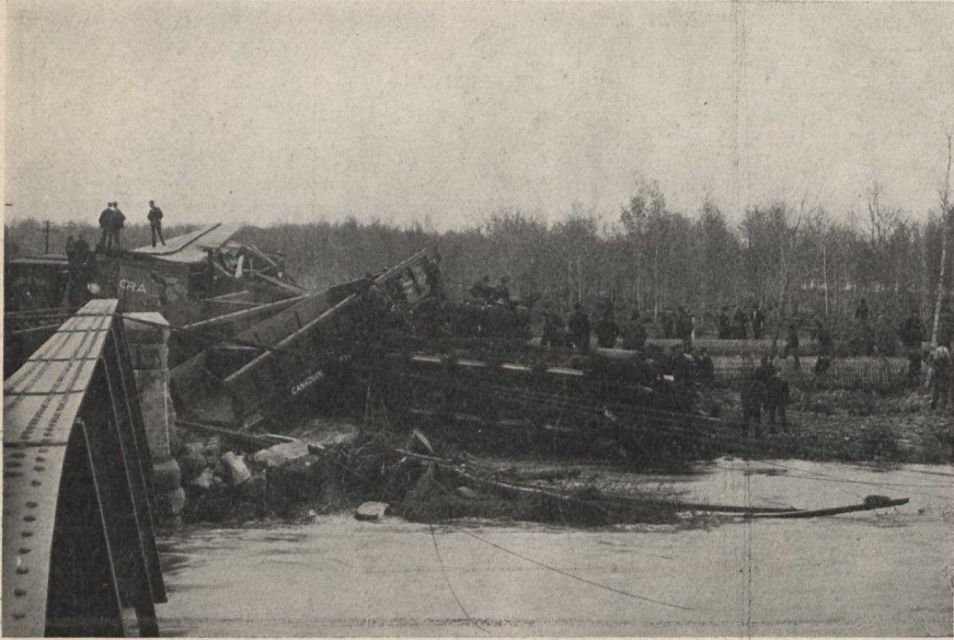
The wreck which caused the death of Engineer Savard, Fireman McBride and Brakeman Inman, at Port Arthur, May 27th.
