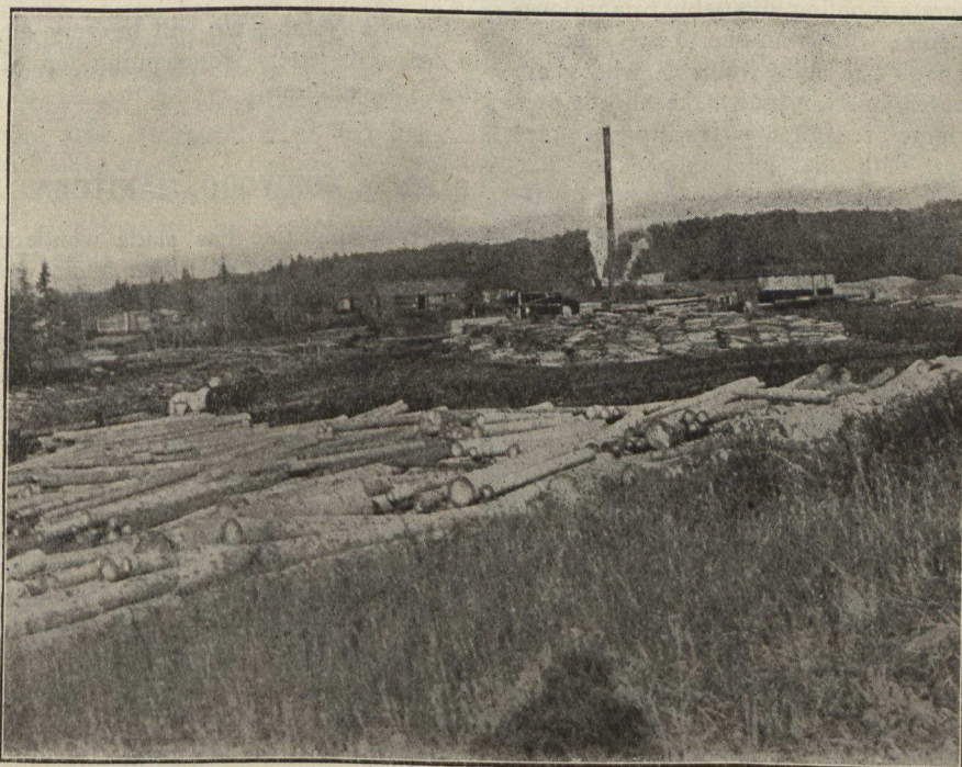
Portable saw-mill on a Dominion forest reserve (prairie provinces) cutting lumber for settlers. As these mills saw only logs cut under settlers' permits this shows how the timber on the reserves is being used to supply the needs of settlers in the neighbourhood.
