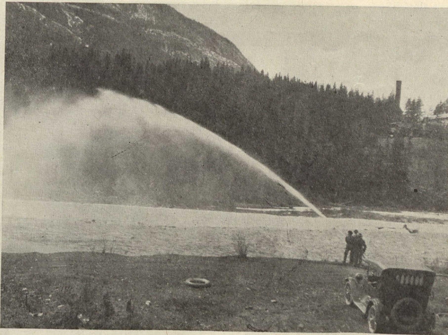
TESTING OUT THE MOTOR FIRE PUMP, BOW RIVER, ALBERTA.
