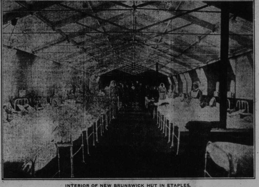
INTERIOR OF NEW BRUNSWICK HUT IN ETAPLES.
