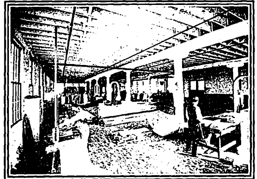
FIG. 5.—ANOTHER VIEW OF GROUND FLOOR OF FACTORY IN WHICH VIBRATION HAS BEEN ALMOST ENTIRELY ELIMINATED BY PLACING THE MAIN SHAFT IN THE BASEMENT, ON CEMENT PIERS BUILT ON INDEPENDENT FOUNDATIONS.
