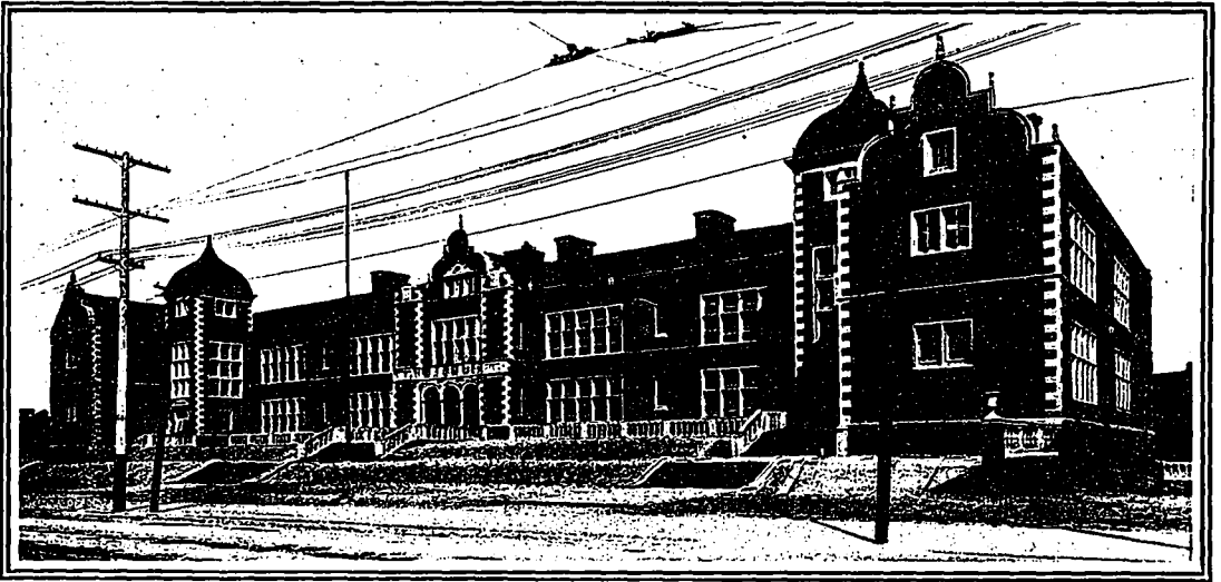
ONE OF THE MORE RECENTLY CONSTRUCTED FIREPROOF SCHOOL BUILDINGS IN ST. LOUIS, MO., KNOWN AS THE WILLIAM CLARK SCHOOL. ARCHITECTURALLY THE BUILDING IS SIMPLE YET DIGNIFIED, AND LENDS AN ATMOSPHERE OF ELEGANCE. BRICK, HOLLOW TILE, CEMENT AND STRUCTURAL STEEL ARE THE MATERIALS WITH WHICH ST. LOUIS SCHOOLS ARE CONSTRUCTED. THIS BUILDING HAS 24 ROOMS, ACCOMMODATING 1,200 PUPILS AND COST $188,902. WILLIAM B. ITTNER, ARCHITECT.
