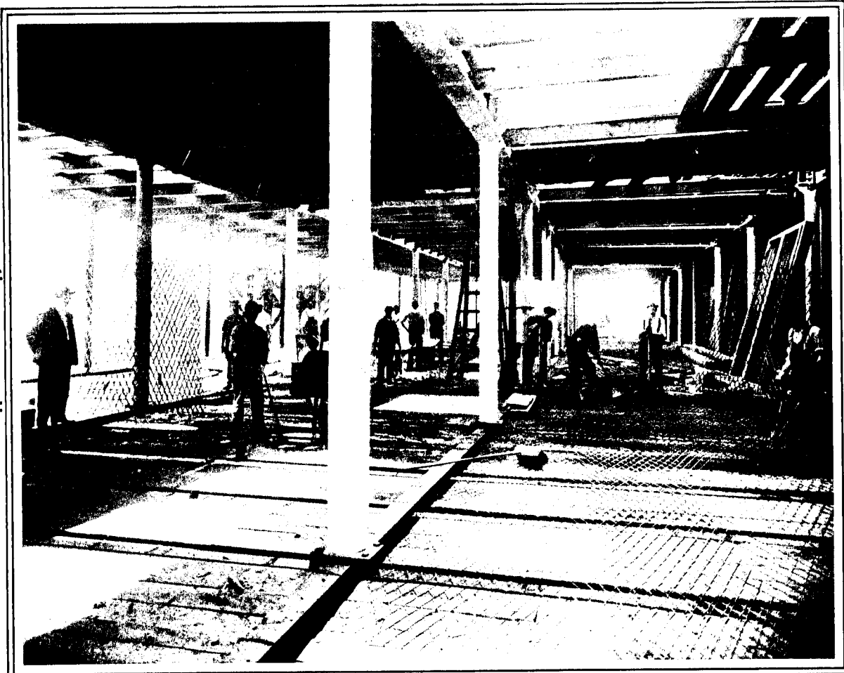
EXPANDED METAL REINFORCEMENT FOR CEMENT FLOORS IN RECENTLY COMPLETED ADDITION TO T. EATON CO.'S STORE, TORONTO
