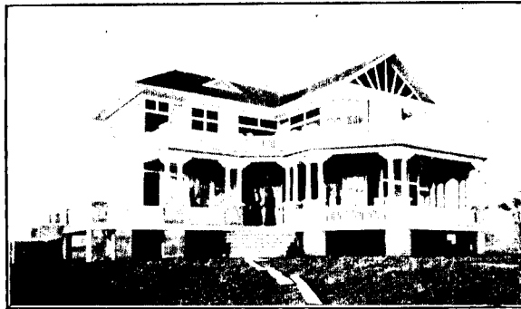
Waterloo County and Country Club House, Galt, Ont. Showing Cement Siding on "Herringbone" Lath, with half-timbered effect.
