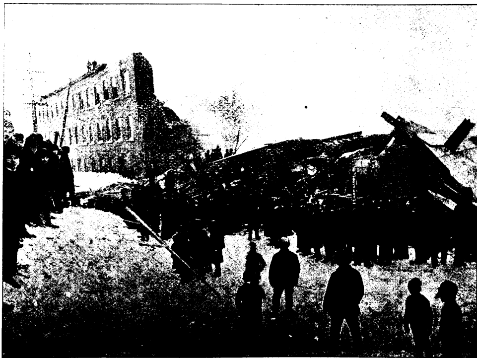
SCENE AFTER RECENT FATAL EXPLOSION IN QUEBEC WORSTED FACTORY.
