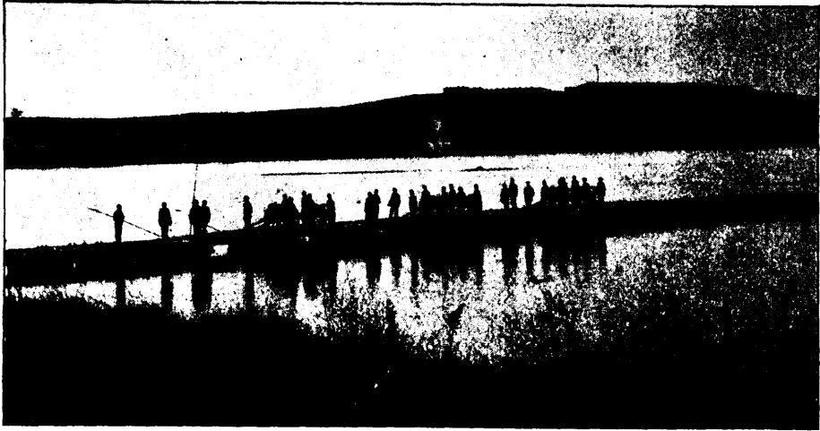
VIEW OF PONTOON BRIDGE, LOOKING TOWARDS FORT HENRY.
