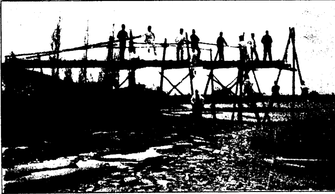
A BRIDGE IN COURSE OF CONSTRUCTION.
