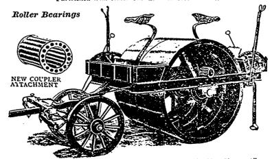
With Roller Bearings and New Patent Coupler Attachment, either 23. 33, 43 or 53 tons. All one size frame, drum, and width of tread and can be extra weighed a tons each. Address for Catalogue
