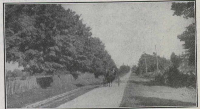
In Wentworth County, on the Dundas and Waterloo Road, Built in 1909.
