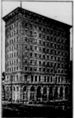
Union Bank Building, Winnipeg
