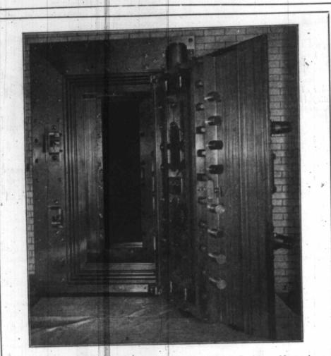
Vault doors in Bank of Montreal and Royal Trust Company, Montreal. Three times larger and heavier than any other in Canada. Doors and Vestibules weigh **60 tons**. Total weight of lining and doors **260 tons**. Accepted to be the finest piece of vault work in construction and workmanship in the Dominion. — Built by the old established firm of
