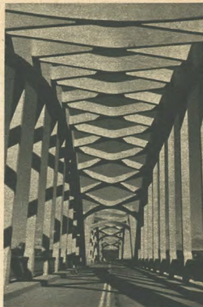
Cement bridge spanning a river in Saskatchewan
