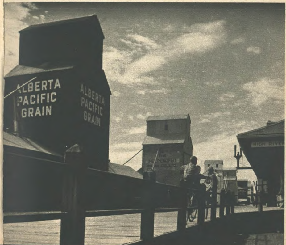
2) Storage silos near Regina, Saskatchewan 3) Grain elevators at High River, Alberta
