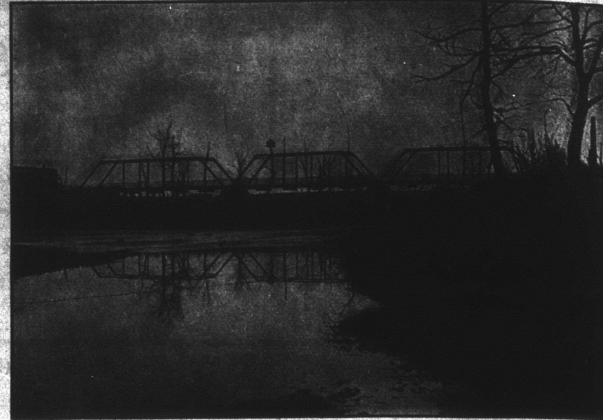
MISSION BRIDGE OVER ELBOW RIVER, CALGARY.
