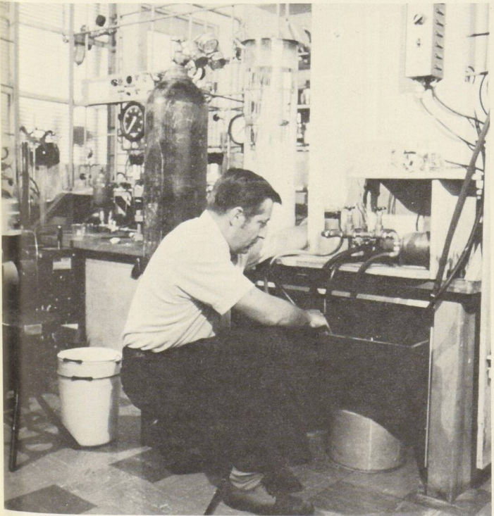
Mr. L. Pageau prepares operating system for casting tubular cellulose acetate membranes.
