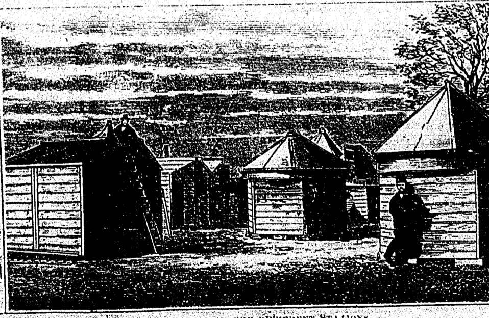
BUILDINGS OF THE DIFFERENT STATIONS.
