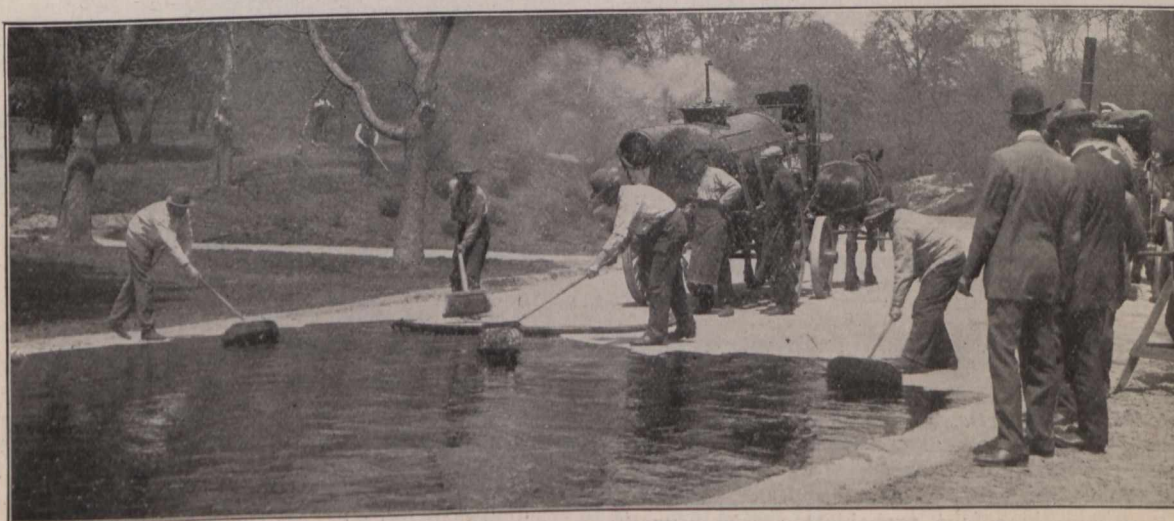
Applying Dolarway Bitumen on Concrete Base, Central Park, N.Y. City.
