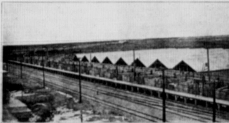
Covered sheds and forty-eight unloading chutes at Winnipeg Stock Yards.
