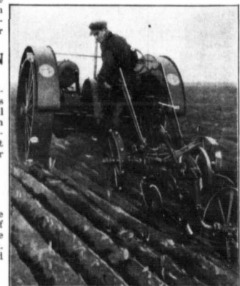
"Happy Farmer" Tractor handling 3 bottom 14 in. Plows, backssetting Timothy Sod at a depth of 8 inches on the farm of Hon. R. P. Roblin, Carman.
