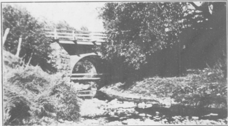
Martin Street Bridge
