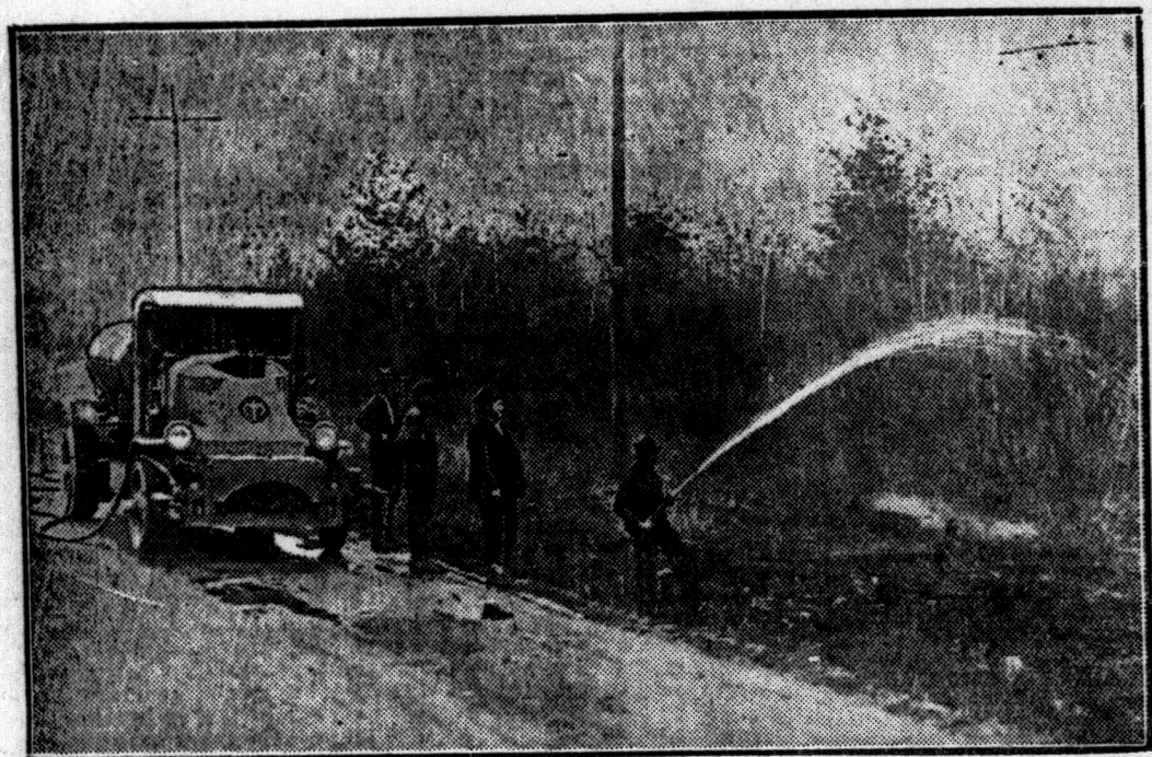
Fighting forest fires in Northern Minnesota. A truck equipped with a chemical tank is driven into the heart of the forest fire district and fights the flames. This is the very newest in combating forest fires
