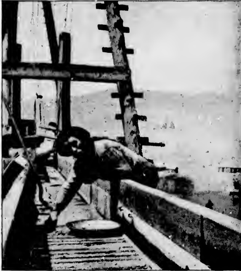
CLEANING UP A SLUICE BOX
