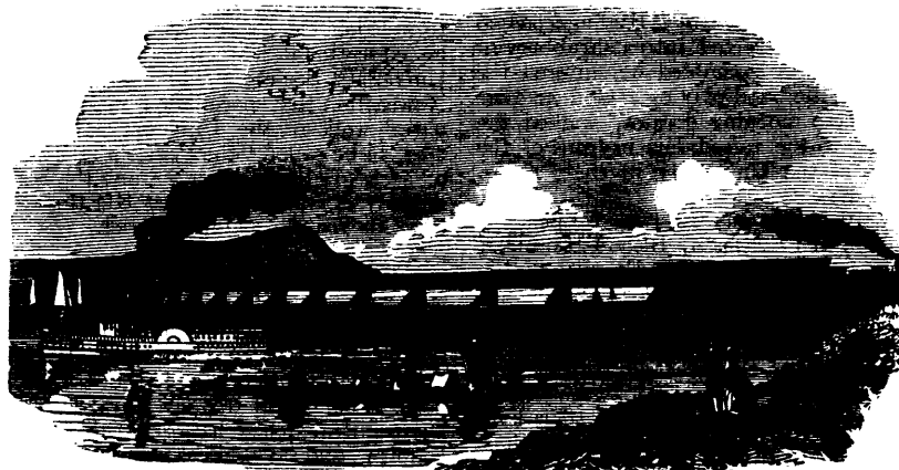
VICTORIA RAILWAY BRIDGE AT MONTREAL, FROM ST. LAMBERT.
