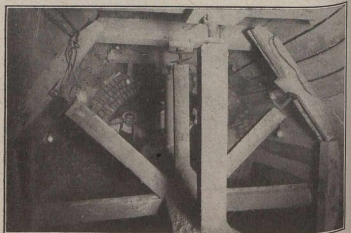
Fig. 7.—Needle-beam Method of Supporting Sheet-piling.
