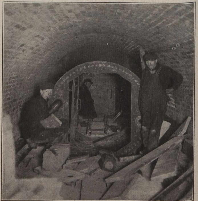
Fig. 4.—Steel Cylinder Air Lock.
