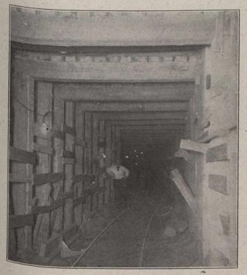
Fig. 8.—Cap and Leg Tunnel.
