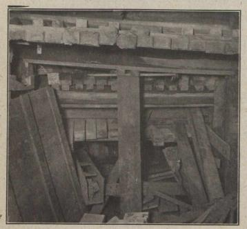
Fig. 2.-Wet Soil Caused Timbering to Sink.
