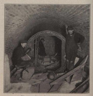
Fig. 4.—Steel Cylinder Air Lock.
