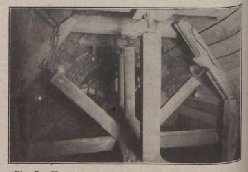
Fig. 7.-Needle-beam Method of Supporting Sheeting.
