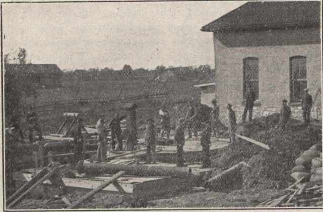
Plant Under Construction.
