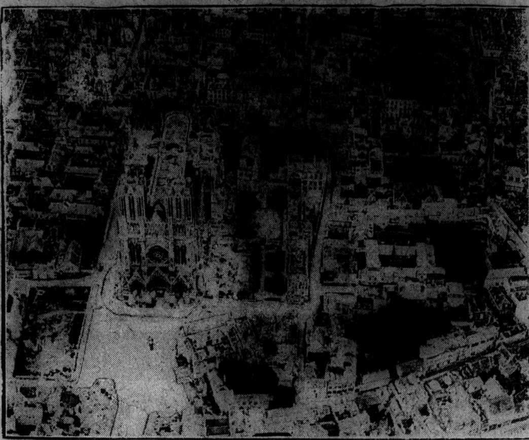
A NEW AIR-VIEW OF THE MARTYRED REHIMS? The martyred town of Reims seen from an aeroplane. The photograph shows the desolate aspect of the section which contains the Cathedral. To the right of the Cathedral are the ruins of the chapel archbishop.
