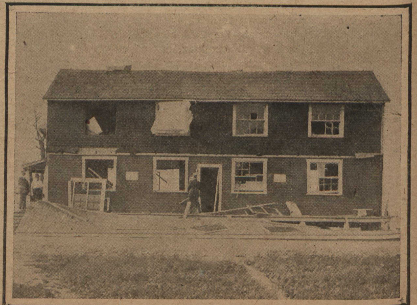
Building wrecked half a mile distant.
