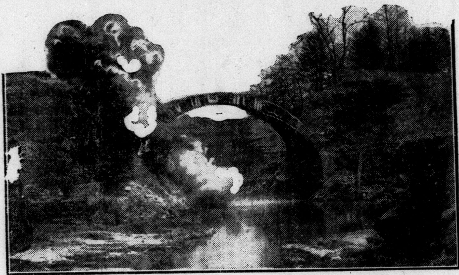
The historic stone arch bridge over the Passaic River at Little Falls, N. J., after standing for more than a century, was blown up recently, to make room for improvements
