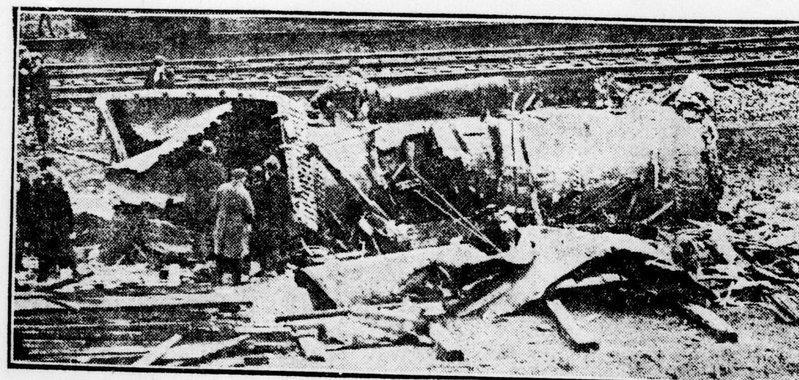
Here is all that is left of a locomotive near Pittsburg recently, when the engine boiler let go, killing the engineer, fireman and road foreman, who was riding in the cab. The train was traveling at 45 miles an hour, but didn't leave the rails
