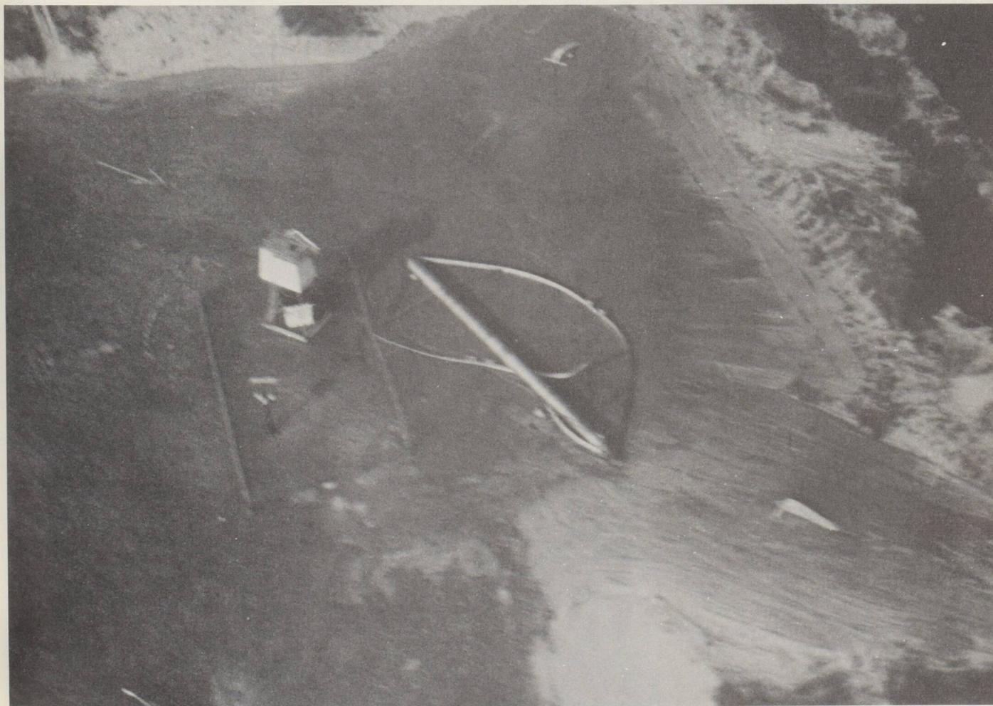
slow evolution experienced a minor revolution in the early decades of this century. Georges Darrieus, a French engineer, patented a completely new kind of windmill. Rather than spinning like an airplane's propeller, around a horizontal axis, its blades curve up and around a vertical axis giving the Darrieus rotor the curious look of a giant egg-beater.
