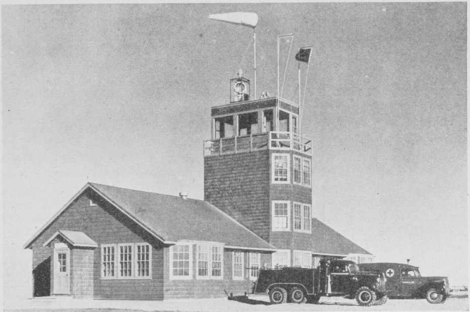
Control Tower. The Fire Engine and Red Cross Ambulance Truck ready for instant use
