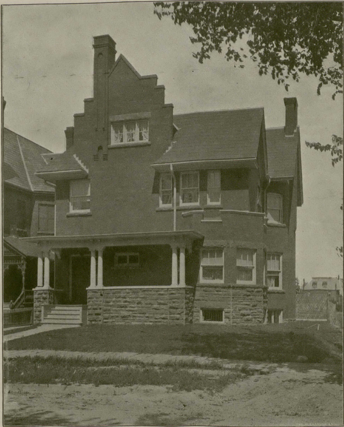
HOUSE ON HURON STREET, TORONTO. MESSRS. SYMONS & RAE, ARCHITECTS.
