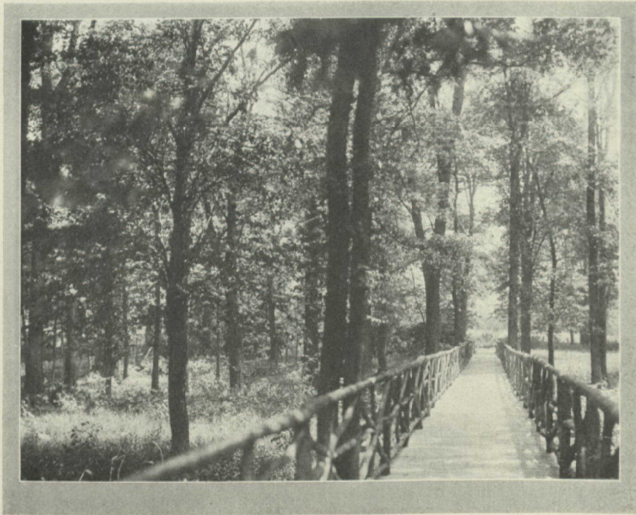
"ELMWOOD." The country residence of Baron Graham at Cartierville. The Viaduct over the Ravine.
