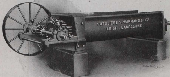
Fig. 1.—Differential Mixer.
