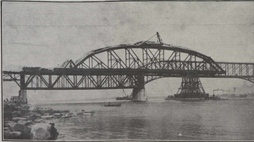
Fig. 1.—Floating One of the New Spans into Position.
