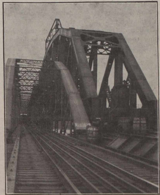
Fig. 3.—View Showing Old and New Spans from the South End.
