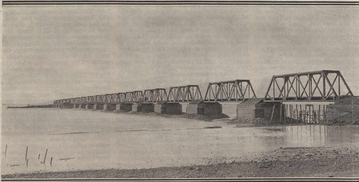
Bridge Pier at Port Nelson, Man.
