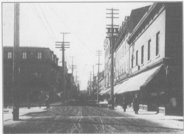
View of Cascades Street looking West.
