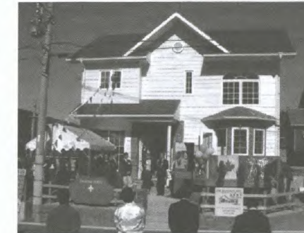
Demtec International's model home at the November 2003 inauguration of its new residential project in Kitakyushu, Japan
