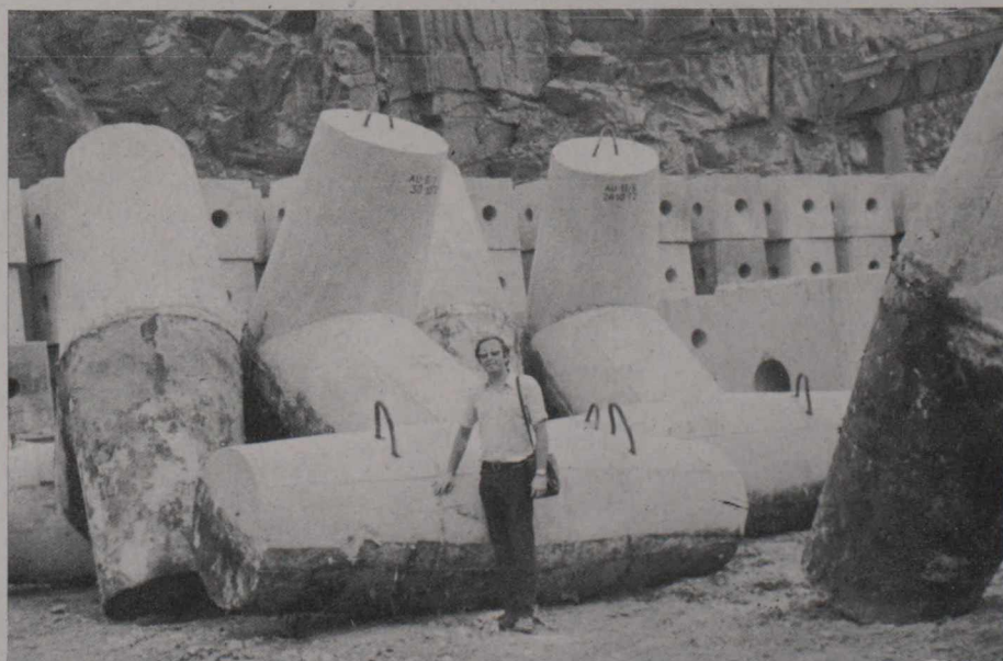
Roessler against the backdrop of concrete tetrapods used at Visakhapatnam
