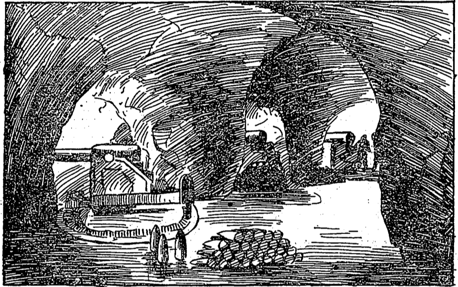
INTERIOR OF BATTERIES.
