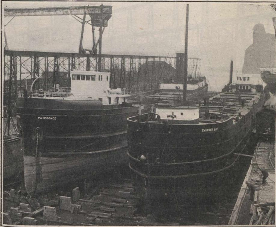
Steamship Paipoonge and Barge Thunder Bay, in Collingwood Shipbuilding Co.'s Drydock No. 2, preparatory to being cut in two to pass through the Welland and St. Lawrence Canals to the Ocean.
