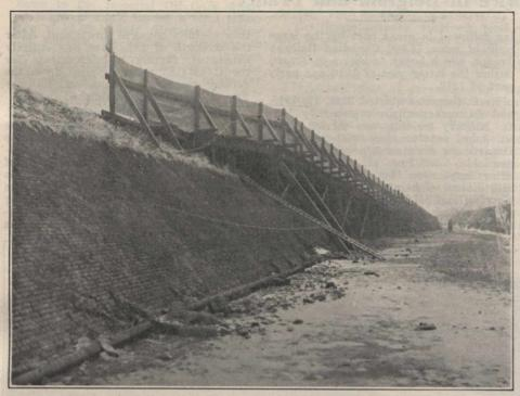
Side view of Timber Ramp, from towpath, to dry bottom of Canal du Nord, to permit it being used as a highway for artillery and team transport. Built by Canadian Overseas Railway Construction Corps, Nov., 1917. The embankment was approximately 40 ft. high.
