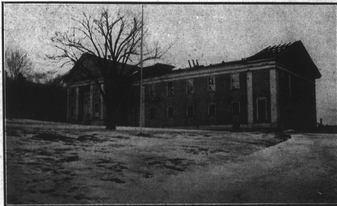
TRINITY CHURCH, HALIFAX. In its ruined state after the explosion of December 6th.
