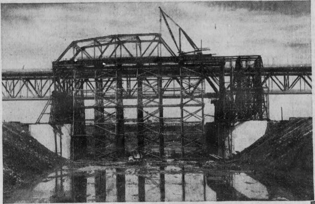
UNIQUE SEAWAY PROJECT is the permanent raising of the southern end of Jacques Cartier bridge, Montreal, and the replacement of one span without interrupting vehicular traffic. This will provide a minimum clearance of 120 feet for shipping in the seaway canal.
