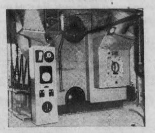
**MODERN TREND IN BOILERS.** Newly developed Dominion Bridge water tube package unit boilers are shop assembled and shipped complete to the site ready for connection to electrical, water and steam lines.
