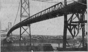
**SUSPENSION BRIDGE IN THE EAST.** The Halifax-Dartmouth bridge, with its main span of 1447 feet and total length of 4420 feet, is the second largest of its type in the Commonwealth—surpassed only by the Lion's Gate bridge, Vancouver, also built by Dominion Bridge.
