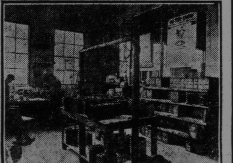
A VIEW OF BATTERY ROOM
