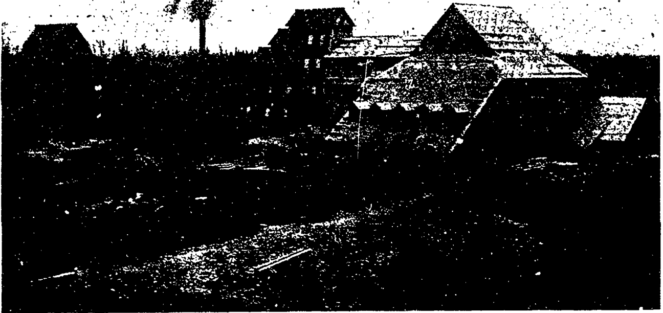
New 60-stamp Battery and Surface Works at Dufferin Mine, Salmon River, Nova Scotia.
