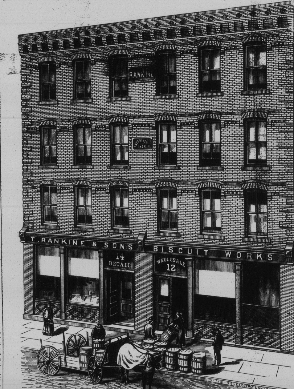
THOMAS RANKINE & SONS' BUILDING.
