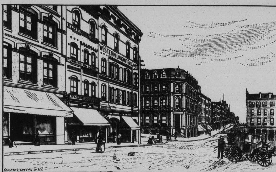
PRINCE WILLIAM STREET, LOOKING SOUTH.
