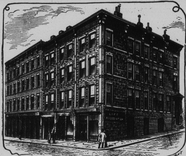
PUGSLEY BUILDING, Cor. Princess and Prince William Sts.
