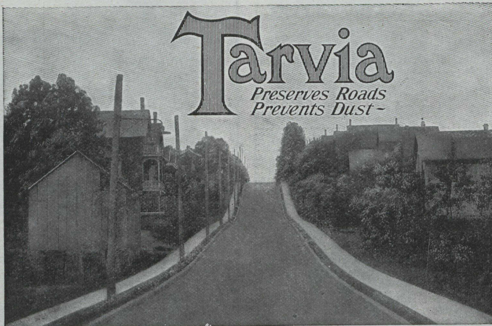
Cedar Street South, Kitchener, Ont. Constructed with Modified Tarvia Modern Pavement.
