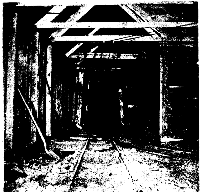
Tunnel No. 3, Ymir Mine.
