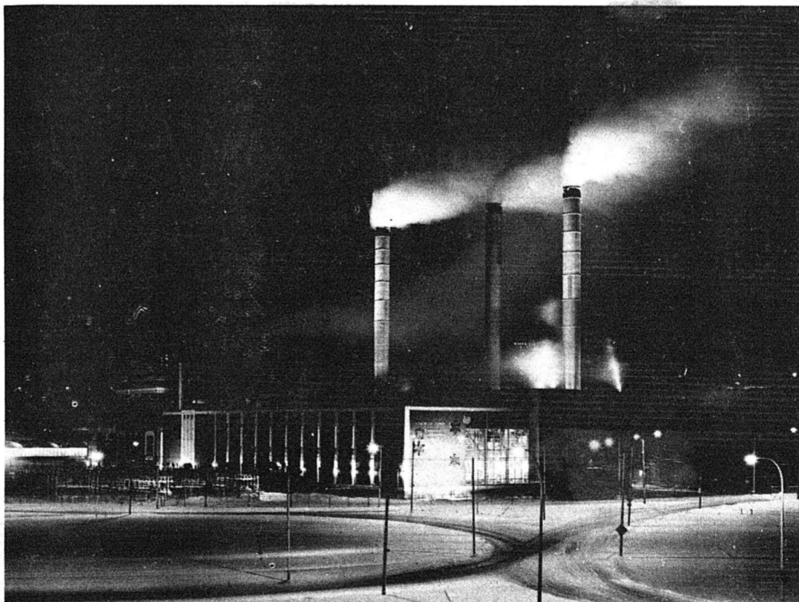
Who would think that a building such as the Edmonton Power Plant could look so beautiful? Photographer Vic Post caught this shot late one night while everyone else avoided the cold.
